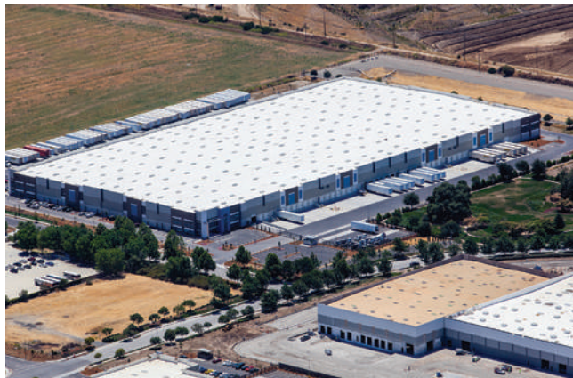
LIVERMORE DISTRIBUTION CENTER, Industrial, San Francisco
