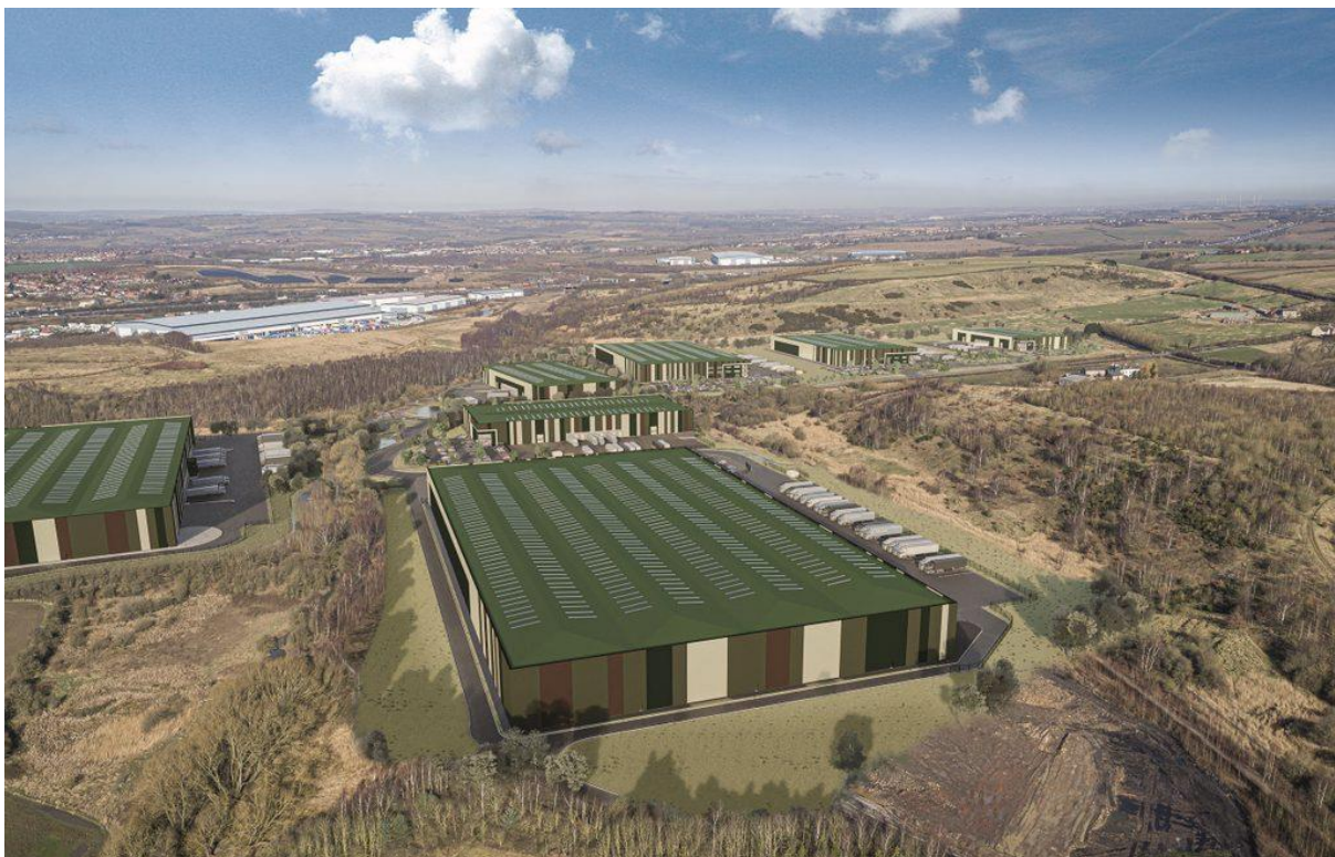
Horizon 29 is the site of the former Coalite works
